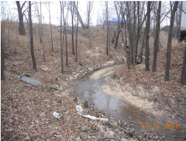
2011 photo looking southwest at the first ditch bend
