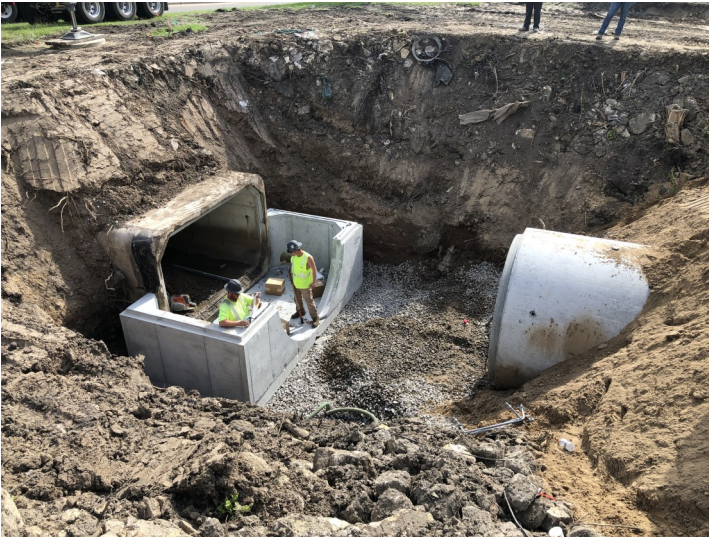
Installation of a box manhole at Terrace Dr
