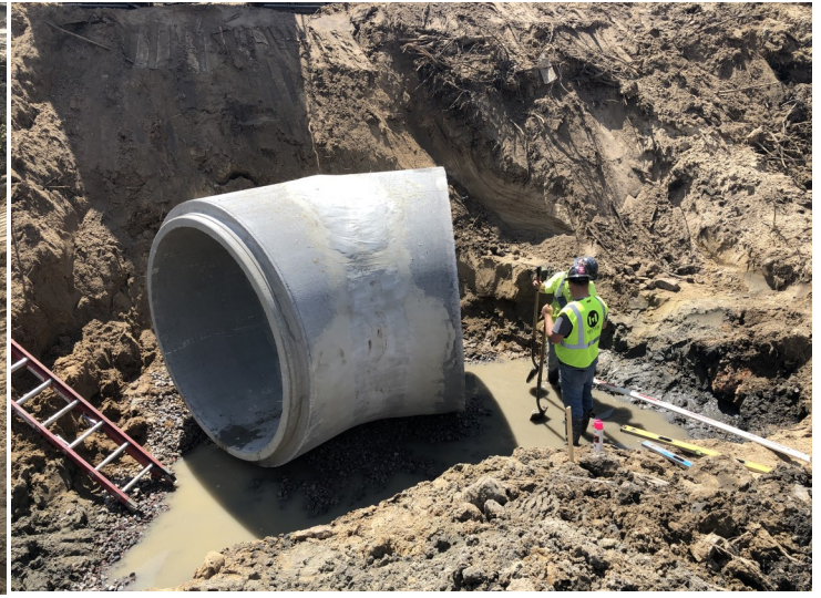
Installation of a bend south of Terrace Dr
