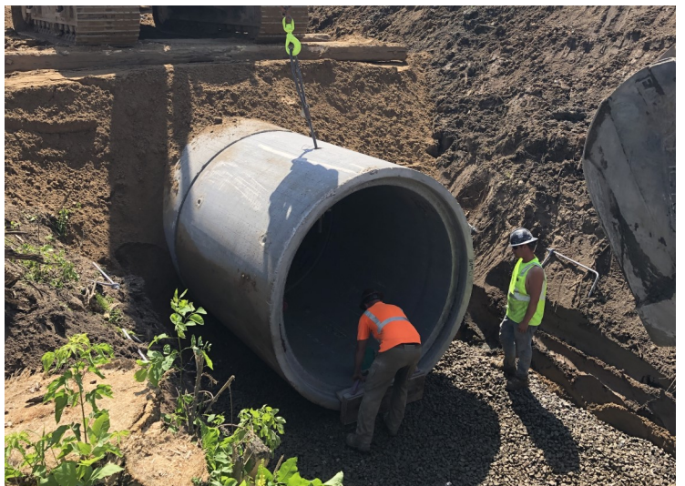
Installation of a section of 84" concrete pipe south of Terrace Dr
