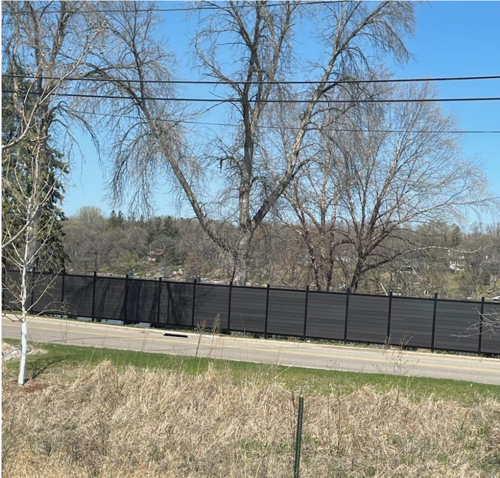
General Appearance of Fence
