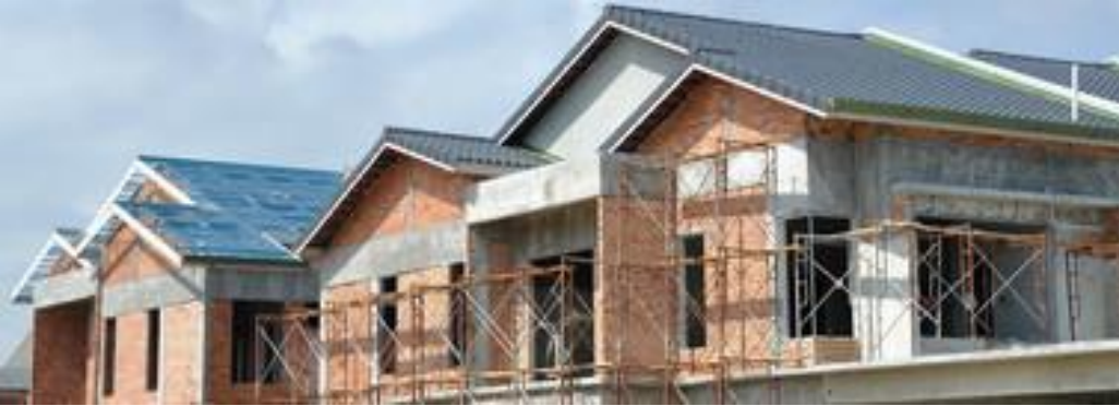
Housing Infrastructure Programs
