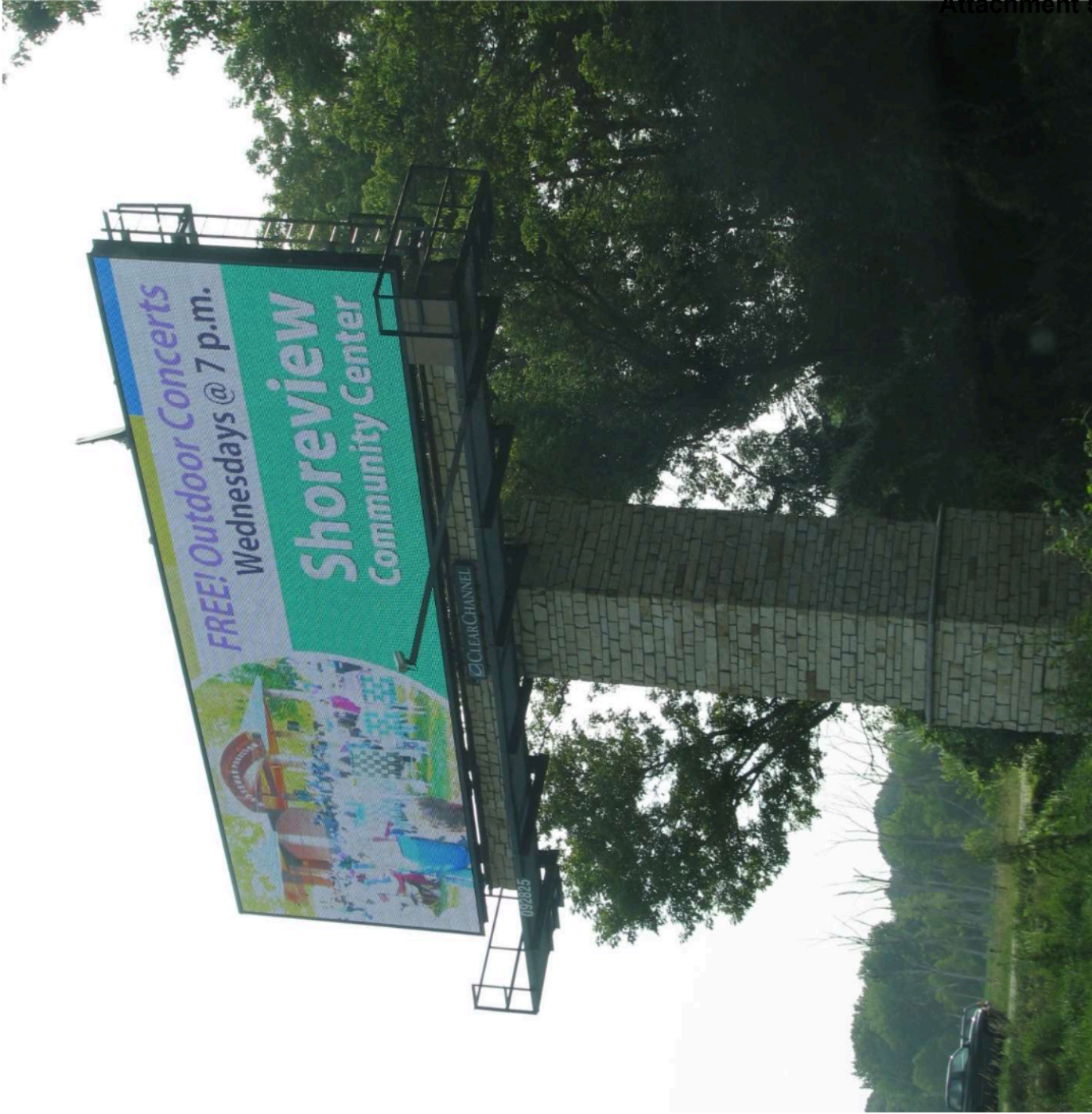
50 ft Tall center mount single face Similar height to St Louis Park Sign - 48ft height
