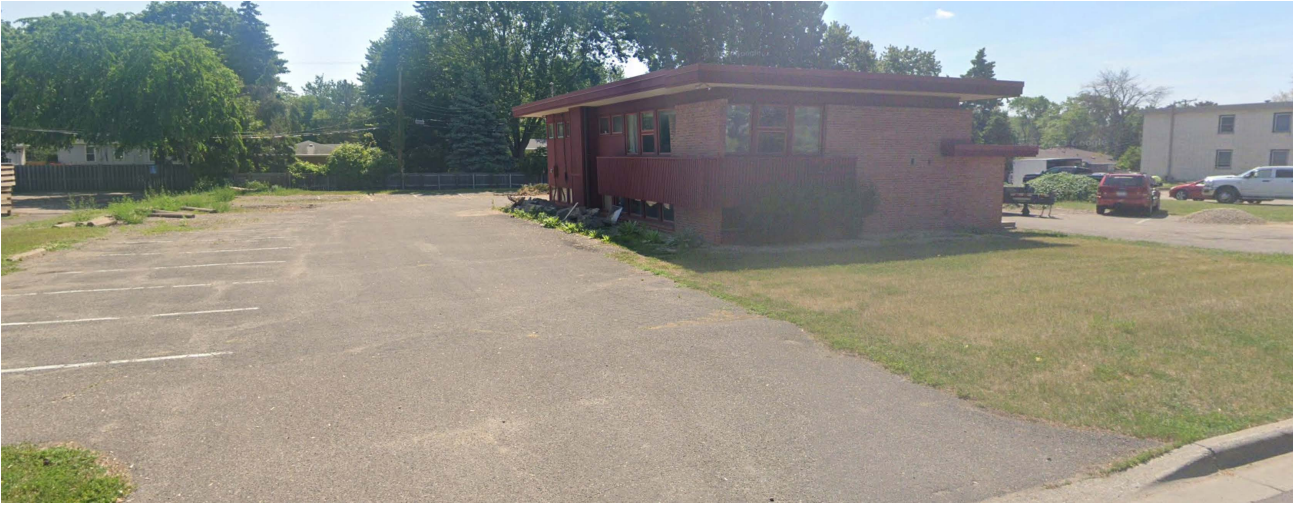
Current building on 2940 Snelling Ave.
