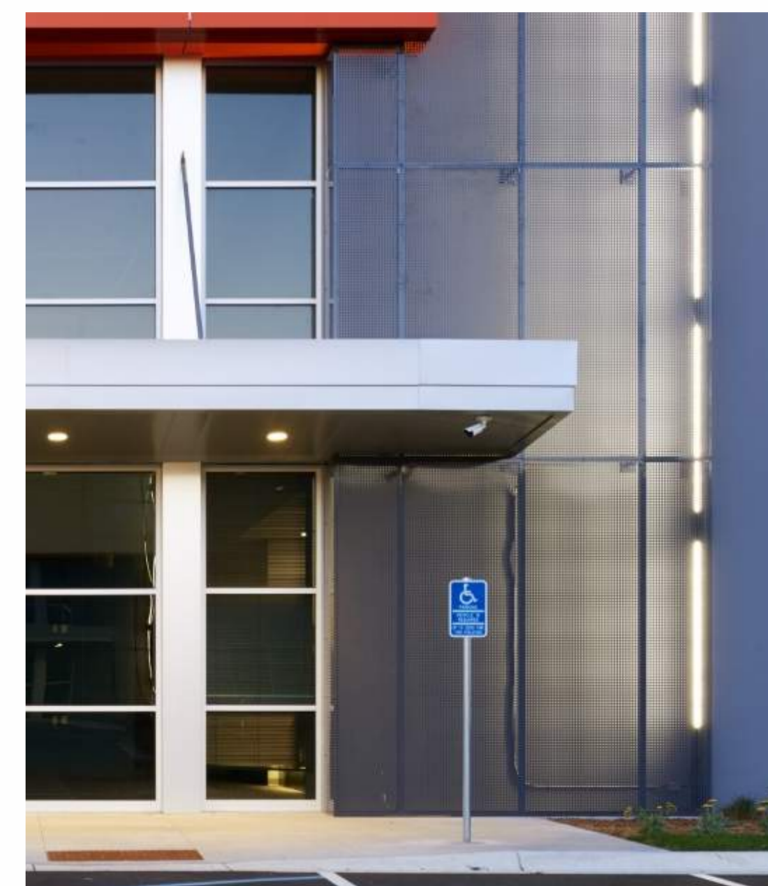
PERFORATED METAL W/ INTEGRATED LIGHTING
