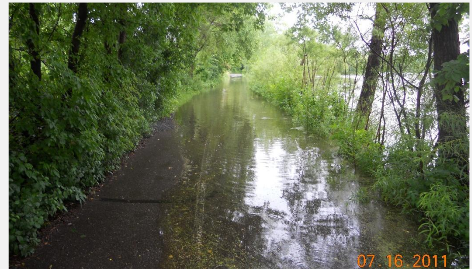
Flooding at Bennet Lake (2011)
