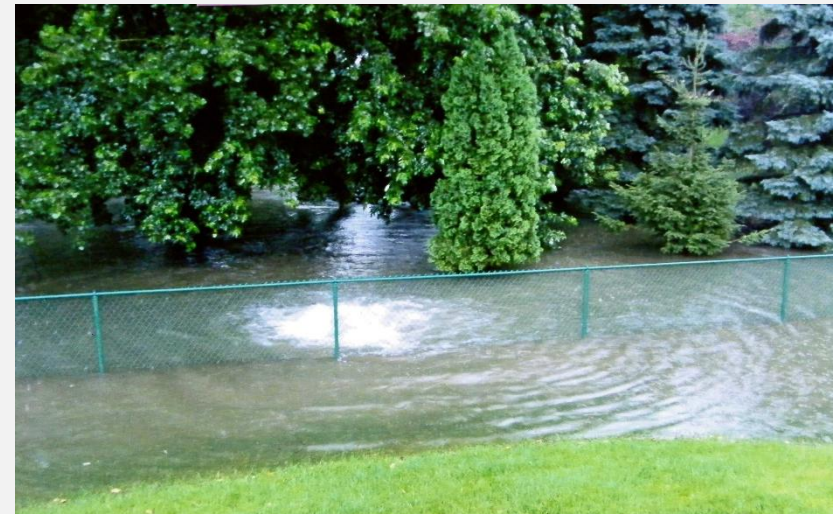
Surcharging (water flowing out) catch basin/manhole
