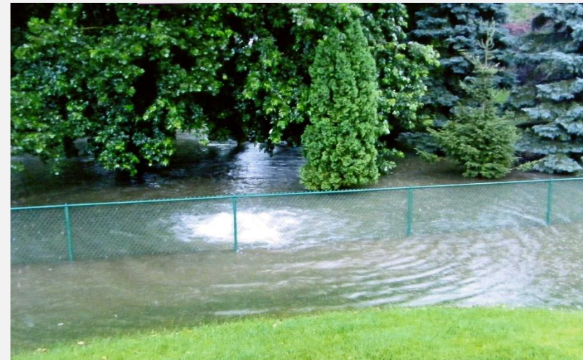
Surcharging (water flowing out) catch basin/manhole
