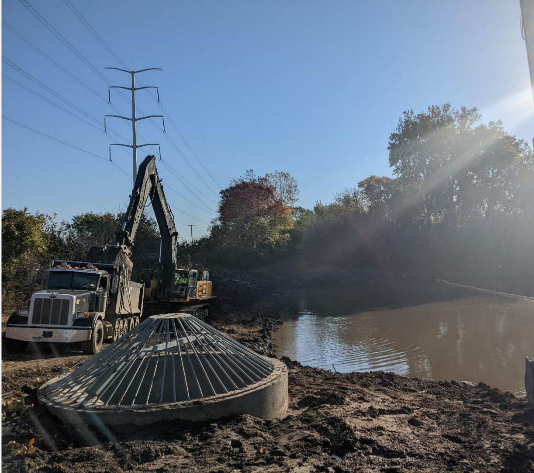
Fairview & C Pond (2022) Post construction
