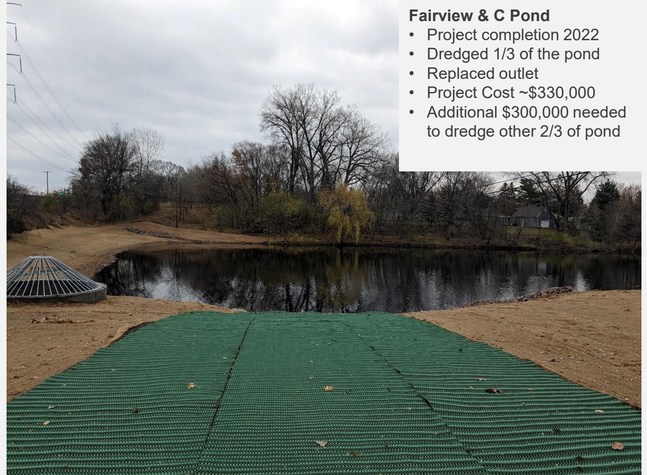
Fairview & C Pond (2022) Post construction
