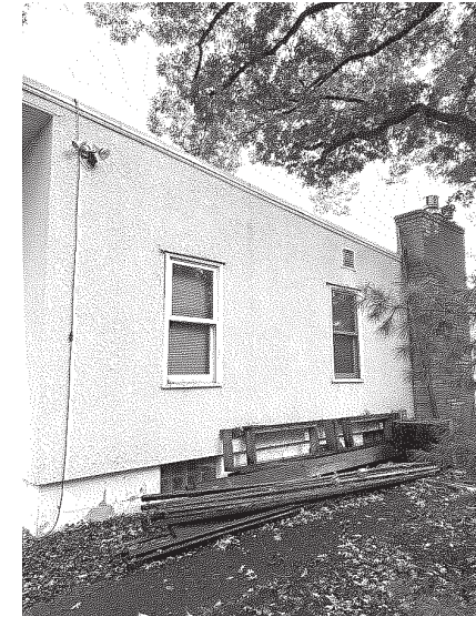
EXISTING CONDITIONS - NORTH VIEW
