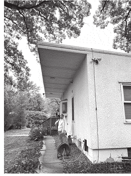
EXISTING CONDITIONS - NORTHEAST VIEW
