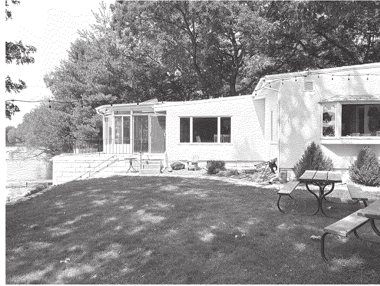
EXISTING CONDITIONS - SOUTH VIEW
