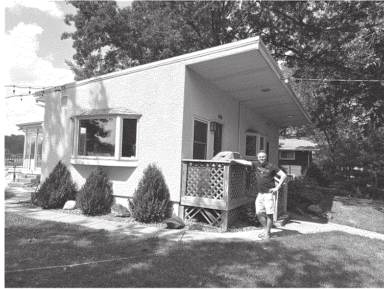
EXISTING CONDITIONS - SOUTHEAST VIEW
