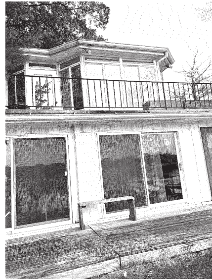
EXISTING CONDITIONS - WEST VIEW
