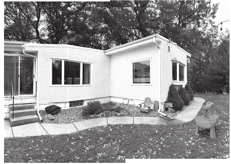
EXISTING CONDITIONS - SOUTHEAST VIEW
