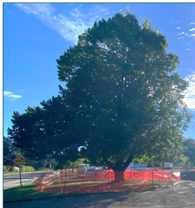
Figure 1- protective drip line construction fencing at Roselawn and Cleveland
